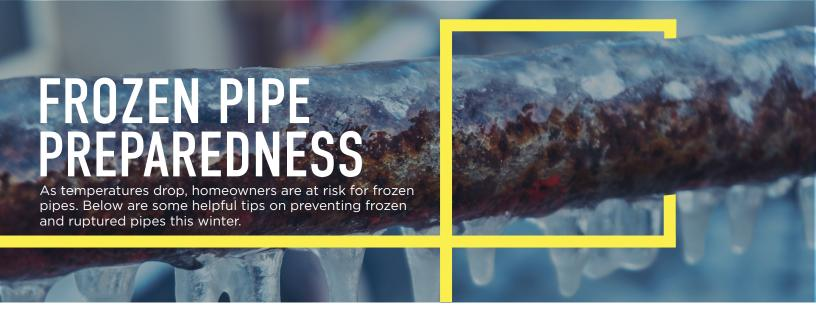
**Let a water faucet drip.** During cold weather, drip water from both hot and cold lines through the system. This will release pressure in the water system, and if the pipes do freeze, dripping water will reduce the likelihood of a rupture.
